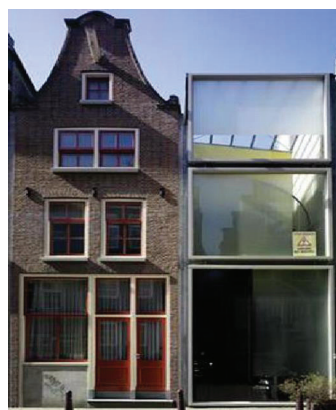
Rooftop-remodeling Falkestrasse, Viena, Austria, Coop Himmelblau, Wolf D. Prix
