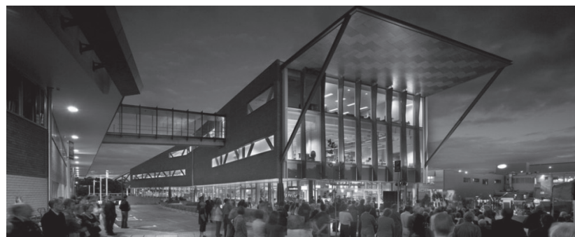
Fig. 16 Biblioteca Waitakere / Waitakere Library , Auckland, Architectus Auckland & Athfield Architects, Noua Zeelandă 2006 http://www.designingfortomorrow.org/images/uploaded/projects/1303121915_large.jpg
