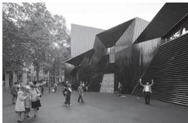
Fig. 10 Centrul comunitar Yesler / Yesler Community Center, Seattle 2005 http://mithun.com/images/projects/1_Yesler_Entry_Masthead.jpg
