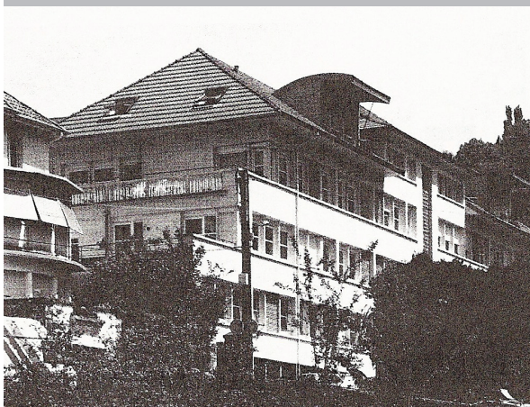
Fig. 7 Imobilul A, reabilitat / Building A, rehabilitated
