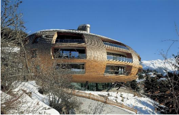
Fig. 13. Chesa Futura – St. Moritz Arhitect: Norman Foster/ Chesa Futura – St. Moritz Architect: Norman Foster. Sursa/Source: fosterandpartners.com © 2023 Foster & Partners © 2023 Nigel Young
