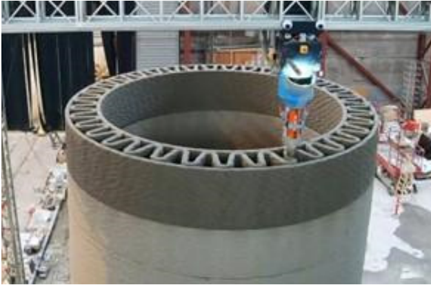
Fig. 4. Imprimarea cu un braț robotic. Sursa: "3D printed wall" by COBOD is licensed under CC BY-SA 4.0/ Printing with robotic arm. Source: "3D printed wall" by COBOD is licensed under CC BY-SA 4.0. Sursa/ Source: https://all3dp.com/1/3d-concrete-printing-guide/
