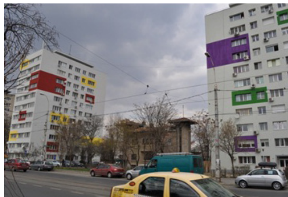
Bloc reabilitat termic, Bulevardul Ion Mihalache / Thermal rehabilitated block of flats, Ion Mihalache Boulevard, Bucharest
