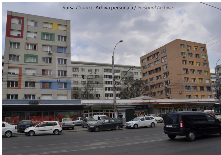
Bloc reabilitat termic, Calea Griviței / Thermal rehabilitated block of flats, Griviței Road, Bucharest
