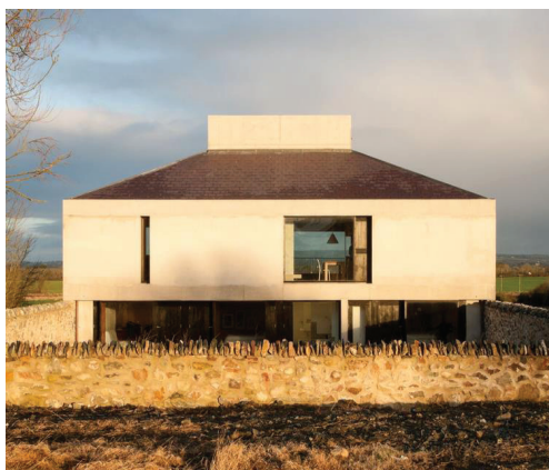
Fig. 5. The House at Bogwest integrată în peisaj cu luminatorul central ieșind din volum./ The House at Bogwest, perfectly integrated into the landscape, with the central skylight standing out from the volume (c) Fotografie: Alice Clancy , Arhitectură: Steve Larkin Architects/ (c) Photo: Alice Clancy , Architecture: Steve Larkin Architects
