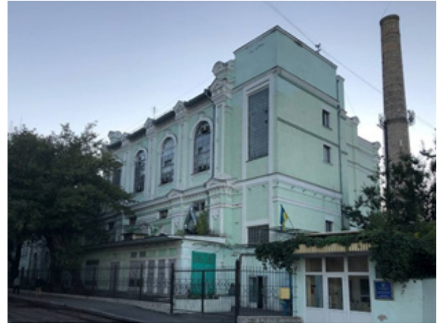
Fig. 4. Complexul Centralei electrice centrale/ Central power station complex Foto/Photo: V. Bonchyk
